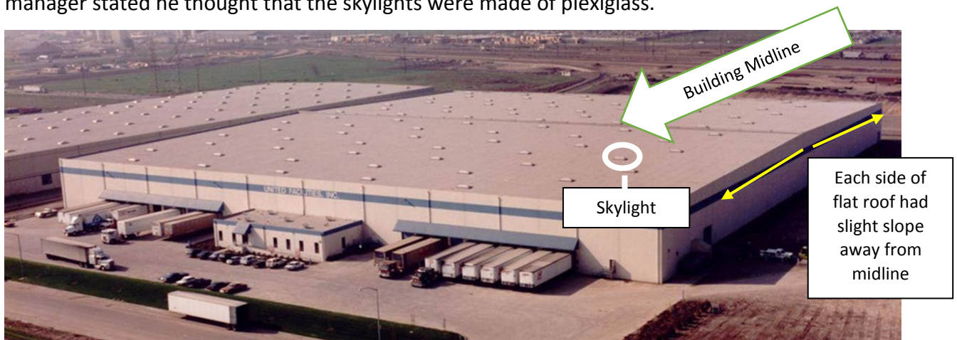
Exhibit 1. The warehouse involved in the incident.
