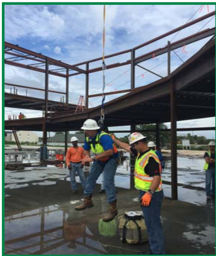
Workers in Louisiana experience what it feels like to hang from the fall protection equipment following a fall.
