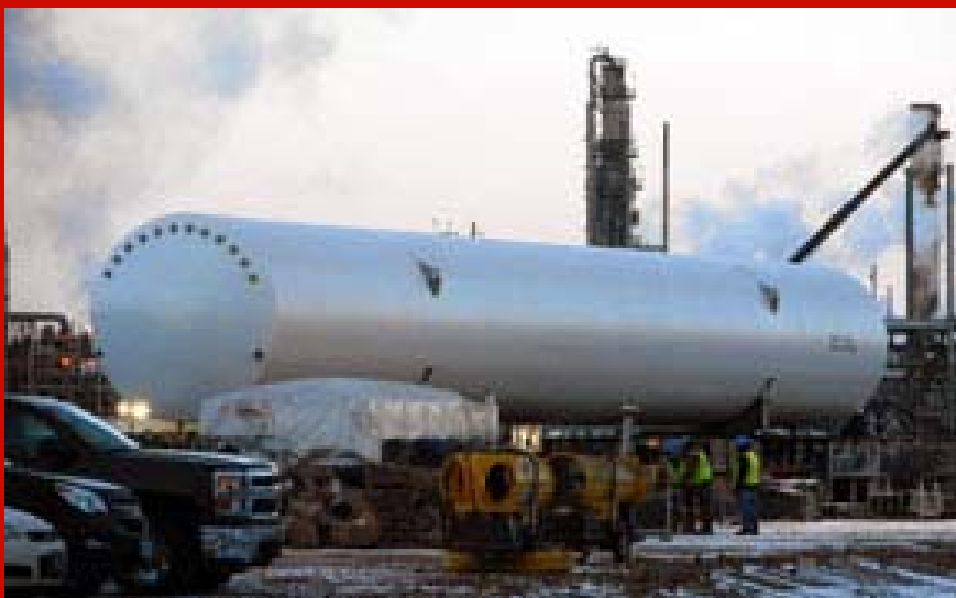
A CO2 tank is delivered to the urea plant project.
