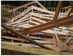
After the 13<sup>th</sup> truss was on the structure and disconnected from the rigging, the system collapsed. Two crew members fell off the top plates and the worker on the floor was struck by a truss and sustained a concussion. The supervisor fell to the floor and was fatally struck by a falling truss.
