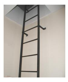
Figure 3 – Example of a roof hatch with a fixed ladder
