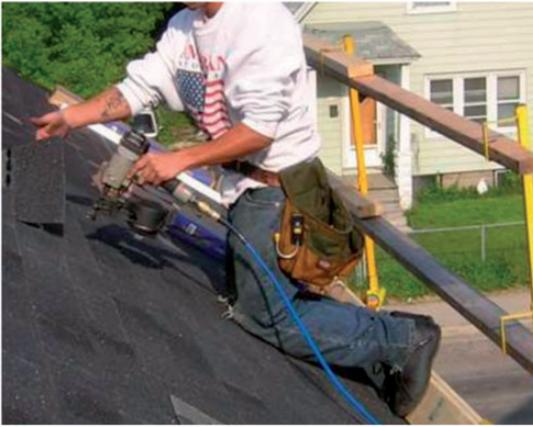
“Got the hand rails up, got the toe boards up (good) pretty safe, and not tied down though. No gloves, but don’t necessarily need it.”
