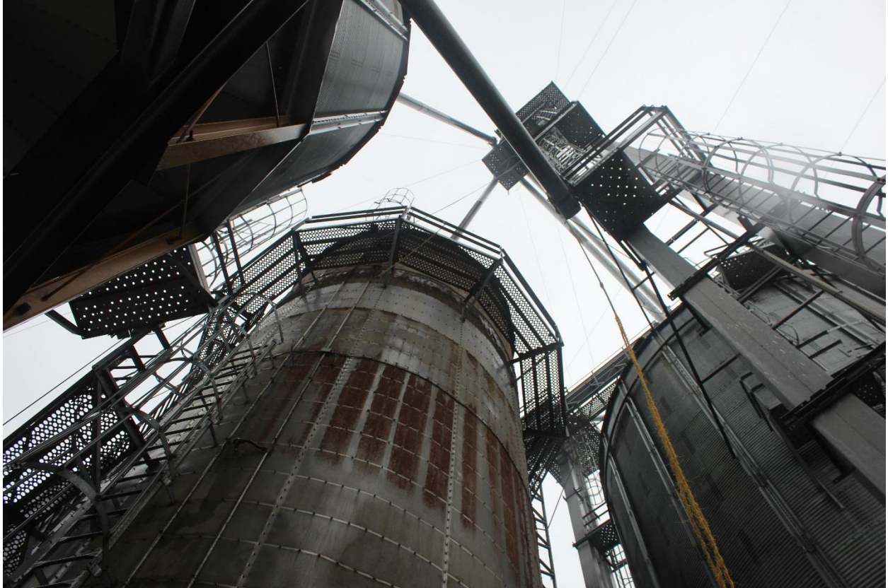
Photo #2 of the grain bin being painted.
