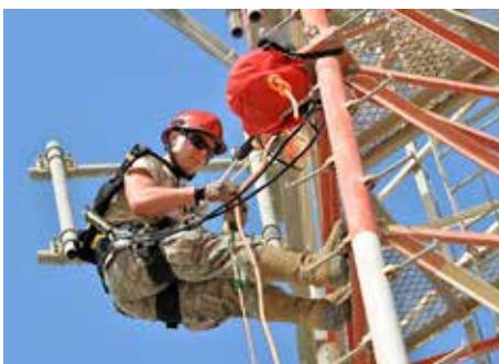
Senior Airman Eric, Cable Maintenance journeyman, climbs a communication tower as part of a demonstration in support of the Air Force fall protection focus initiative at an undisclosed location in Southwest Asia May 11, 2015. According to the Air Force Safety Center website, the Air Force experiences hundreds of fall mishaps annually that result in thousands of lost man-hours as well as injuries and deaths.
