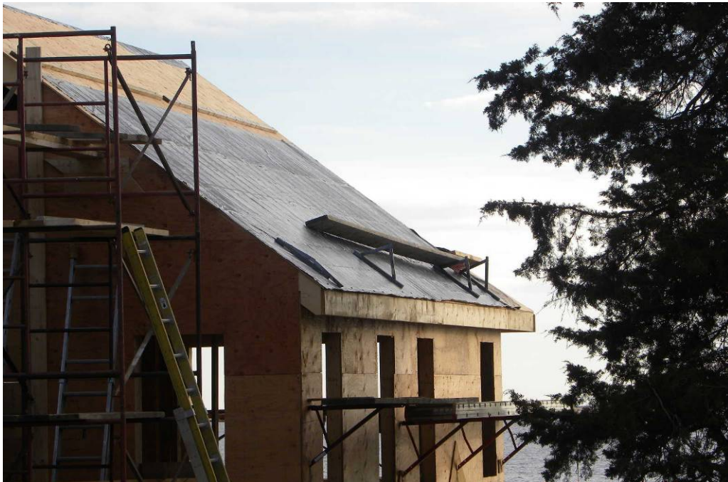
Figure 3 – Roof with roof bracket folded flat
