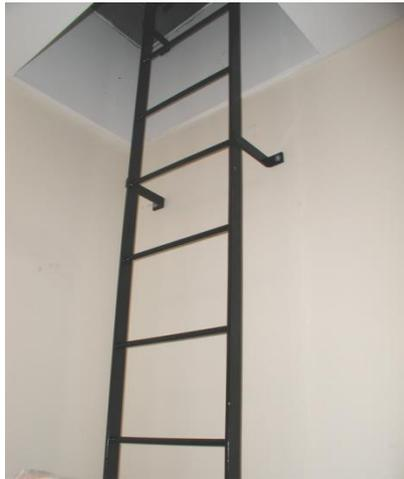
**Figure 3 – Example of a roof hatch with a fixed ladder**
