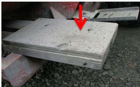
Figure 2. Close-up of wooden platform constructed by employer.
