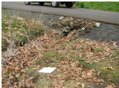
Figure 4. Landscape culvert and sloped surface on edge of roadway traveled.
