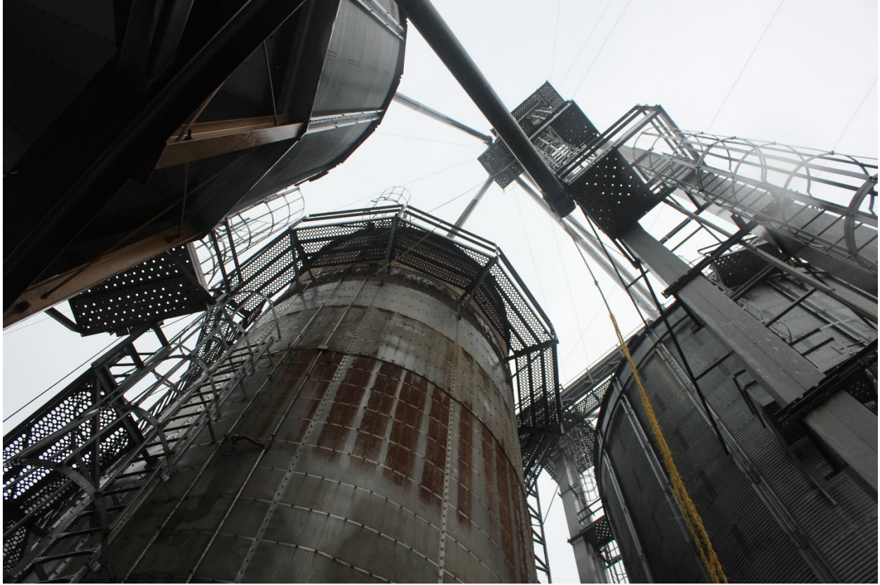
Photo #2 of the grain bin being painted.
