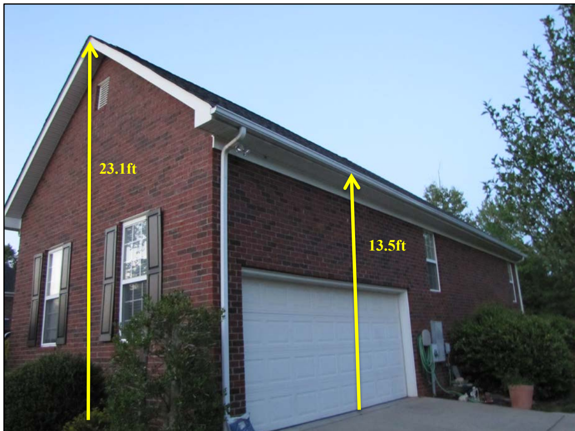
Photo 2. Garage where laborer was working (Photo courtesy of NCDOL/OSH)
