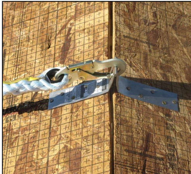
Photo 7. Proper installation of PFAS anchor (Photo courtesy of NAHB) 7
