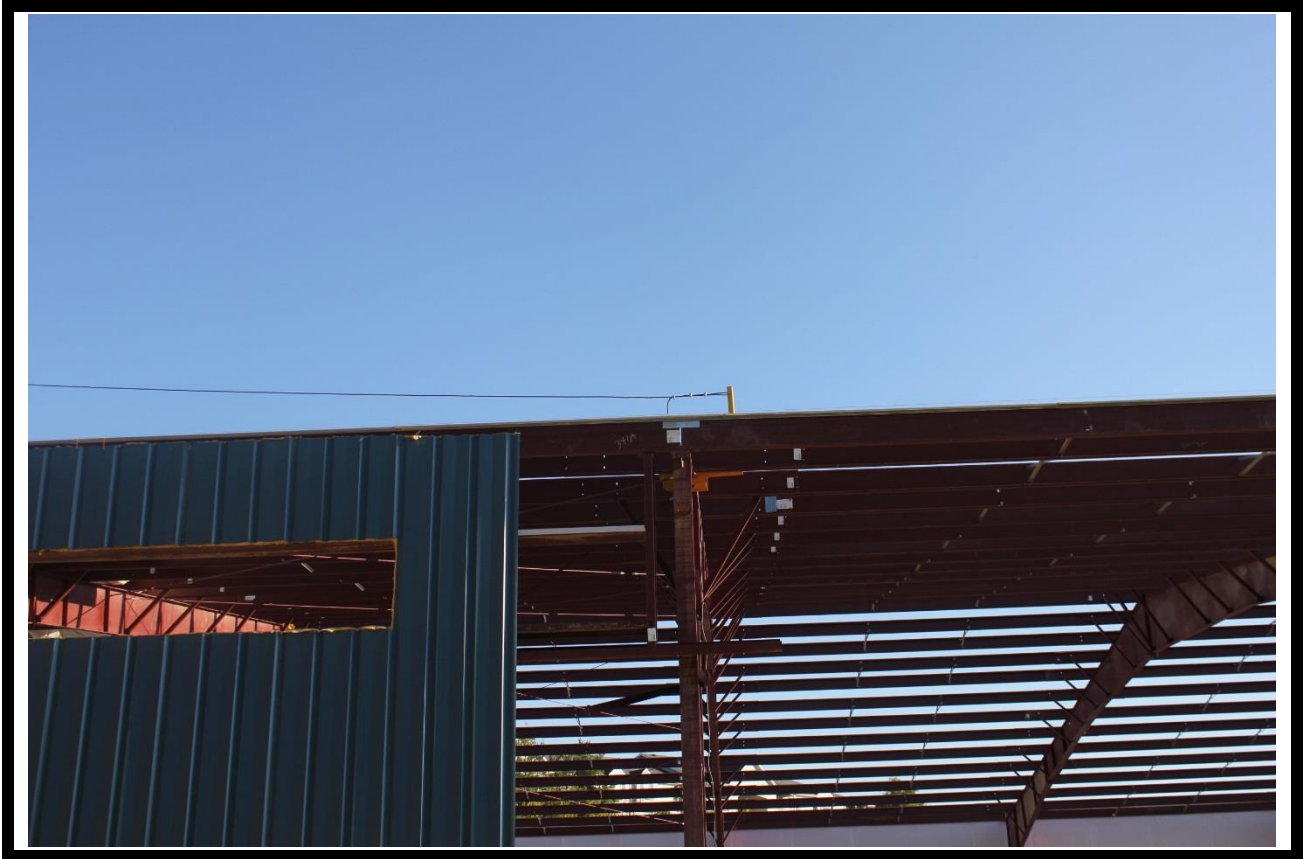
Picture of the steel building with zip line tie-off point. Photograph courtesy of KYOSH
