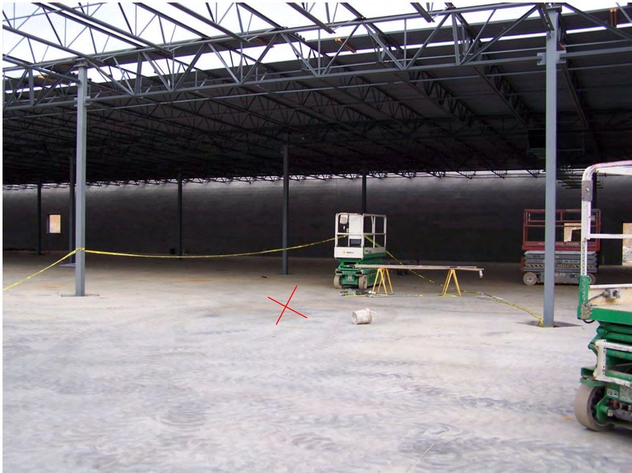
Location where foreman fell.
