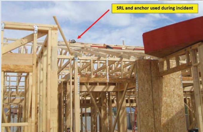
Photo 2: PFAS anchor and SRL used by the worker. All equipment left in place for photo.
