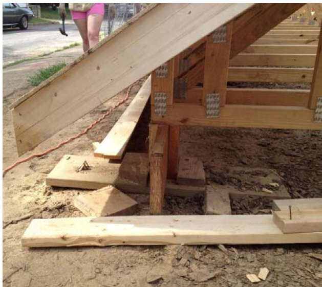
Figure 11 – Roof assembly built on stationary base.
