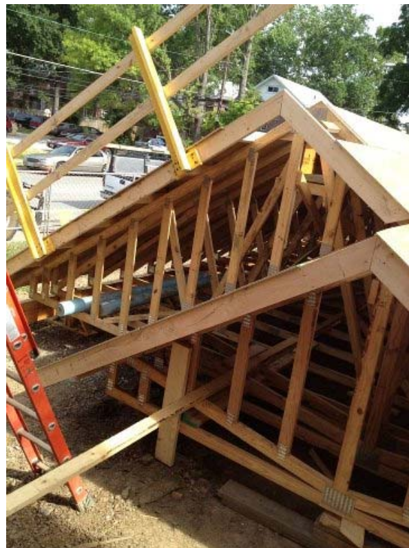
Figure 12 – Guardrail protects the gable end of truss.
