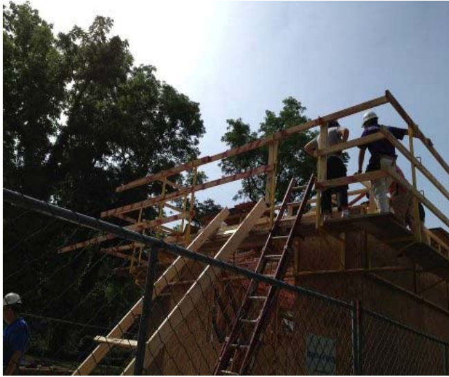
Figure 5 – Hanging scaffold system in place.
