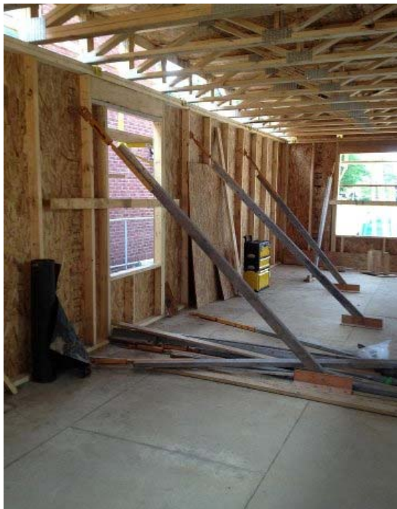
Figure 7 – Interior bracing supports scaffold and workers (right).
