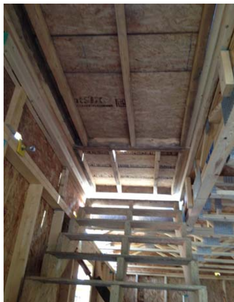
Figure 10 – Stair covers in place from below.
