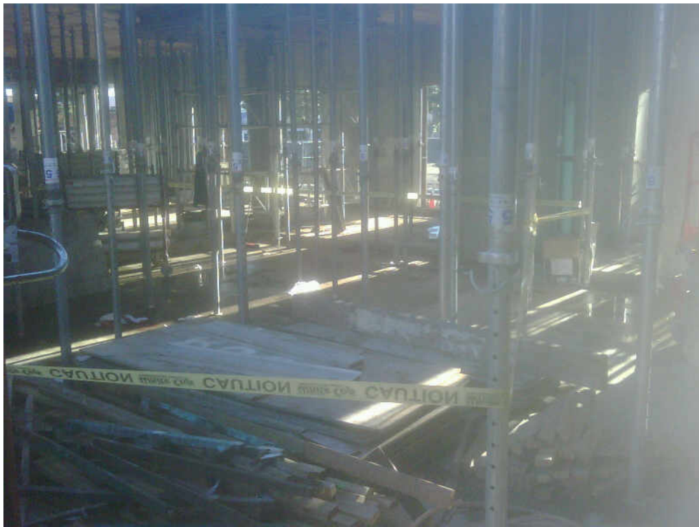
Exhibit 5. The vertical shoring and the support post.
