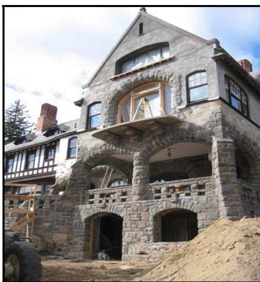
Photo 1 Second story addition (courtesy of OSHA)
