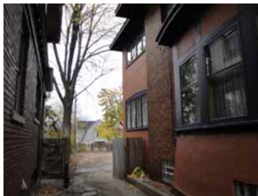
Figure 1. Overview of incident scene
