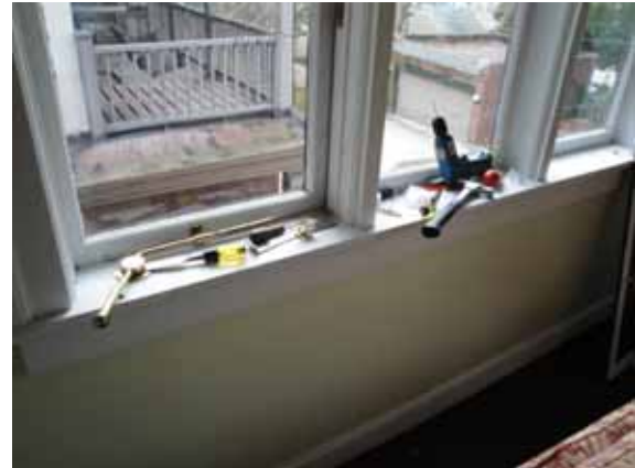
Figure 2. Work performed inside of home
